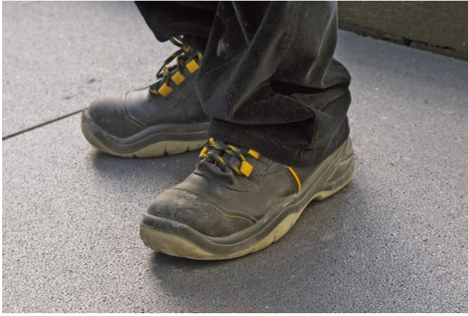
Fig. 4. Stable insulation boards are the preferred material for utilised single-layer flat roofs, since they show no deformation, even under high loads.
