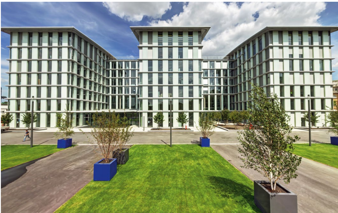
Fig. 5. In addition to conference rooms and a modern staff restaurant, the new BASF office building D105 in Ludwigshafen offers multi-functional office spaces for 1,200 employees
